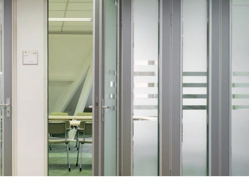
Each wall section incorporates an end pass door panel, which provides a quick method of closing off the wall and also a means of access into adjoining rooms.
